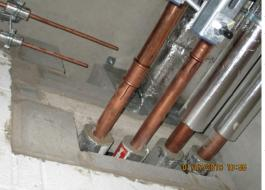
BWK hole with multiple service penetrations, where additional blockwork and lintel had to be installed retrospectively to achieve a 'standard' installation.
